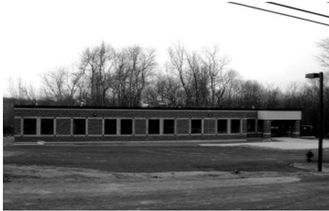
The new MHG Central Office (shown here in a construction photo) is located at 35 Avco Road, Haverhill.
